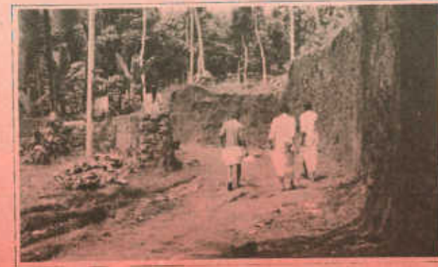
Mangattu Kavala, Newman College Road Under Construction
