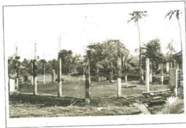
College Chappel under Construction
